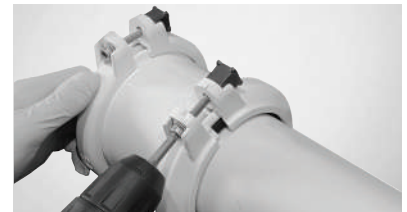
3 Clamp tightening (an electric drill) and finishing
