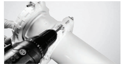
③ Clamp tightening (an electric drill) and finishing
